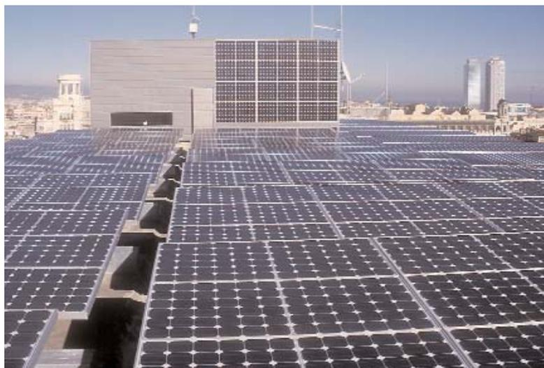
One of the emblematic solar energy facilities in Barcelona is the photovoltaic pergola placed on the roof of the main City Council buildings. Its power is 85 kWp, its collectors take up 650 sqm and it generates 93,000 kWh every year, which implies that almost 10 metric tons of CO<sub>2</sub> emissions are avoided.
